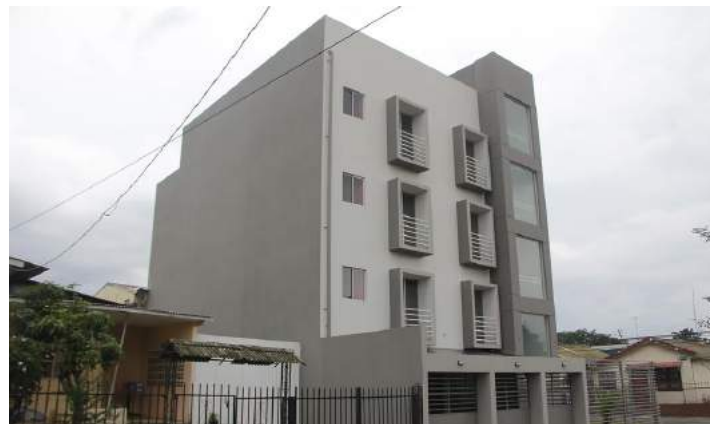
02_Image: Photograph of main facade / Fotografía Exterior fachada principal
