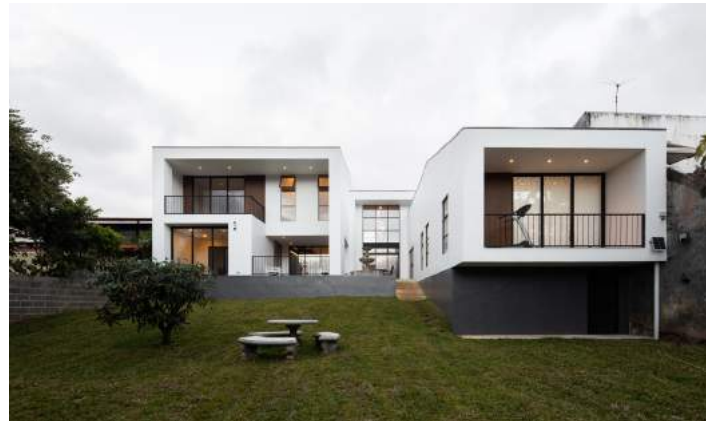
03_Image: Photograph of rear facade (morning) / Fotografía de fachada posterior (dia)
